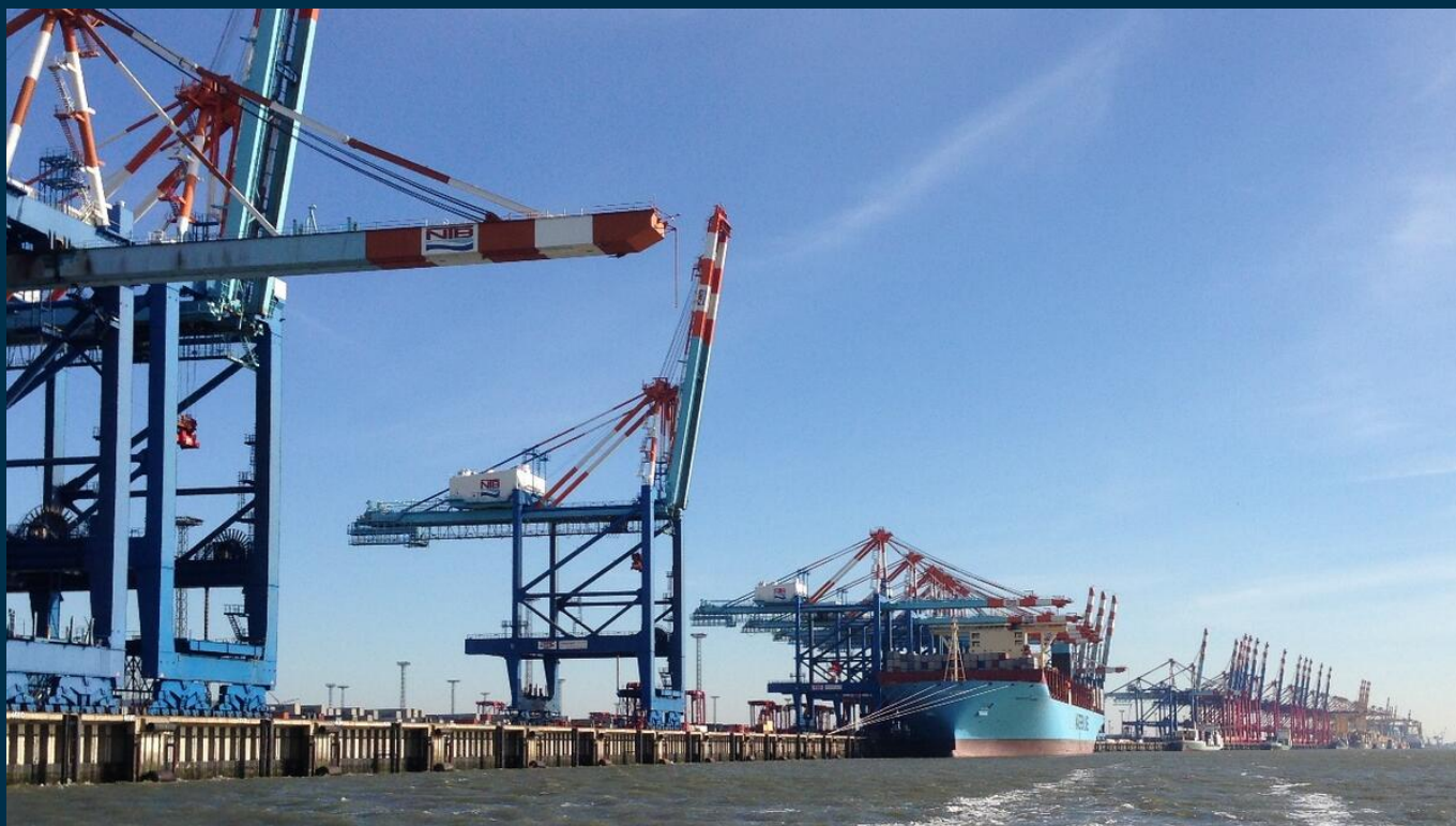
Photo: CWSS/ Bostelmann. Container terminal in Bremerhaven (DE).
