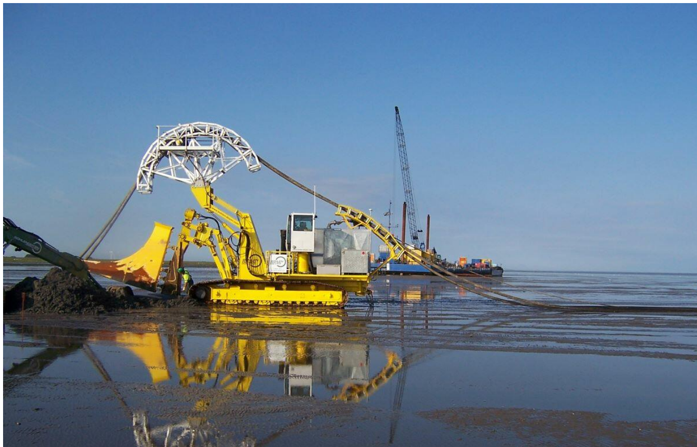
Figure 10. The vibration cable plough is a laying tool utilized for tidal flats (Source: Bohlen & Doyen).
