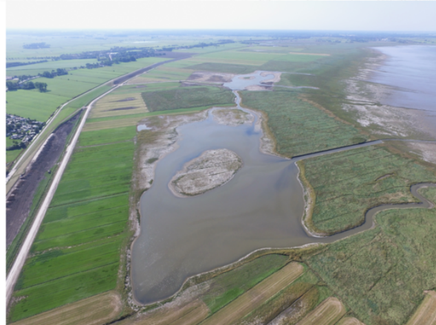
Figure 15. Example of re-designing and rewetting an artificial salt marsh after clay extraction by removing the top soil in the Neuwapeler Außenroden, Jadebusen, Lower Saxony. The photo shows the re-designed sections A and B (90° rotated). (Photo and schematic overview: Planungsgruppe Grün, Herr Sprötge; legend translated and modified by the authors).
